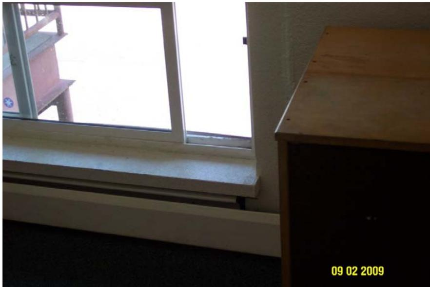
**Photograph 2 – Taken at the Bemis facility on 9/2/2009 showing a classroom window located above the baseboard heater and accessible to children but without a guard to prevent a child from falling through the screen.**
