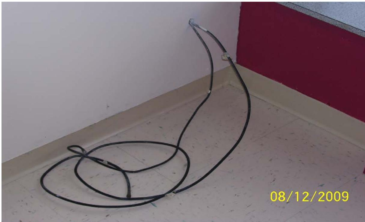
**Photograph 6 – Taken at North Fond du Lac on December 8, 2009, showing loose wires coming out of the wall in an area accessible to children.**
