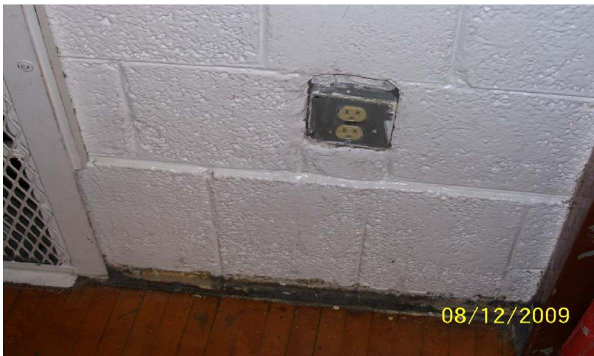
**Photograph 3 – Taken at North Fond du Lac on December 8, 2009, showing an electrical outlet in the gymnasium without a safety cap.**
