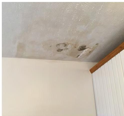
**Photograph 4: Water damage and mold.**
