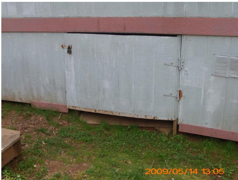
**Photograph 2 – Taken at the Haralson County facility on 5/14/09 showing an exterior door panel that did not extend to the ground, allowing children to crawl under the door.**
