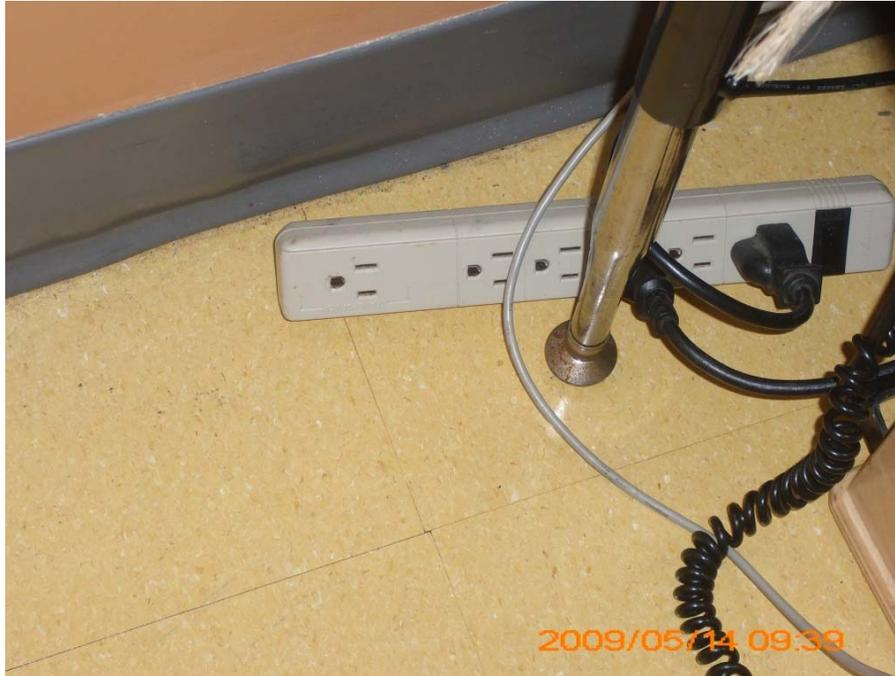
**Photograph 3 – Taken at one Paulding County facility (Hiram YMCA) on 5/14/09 showing multiple electrical outlets without protective caps.**
