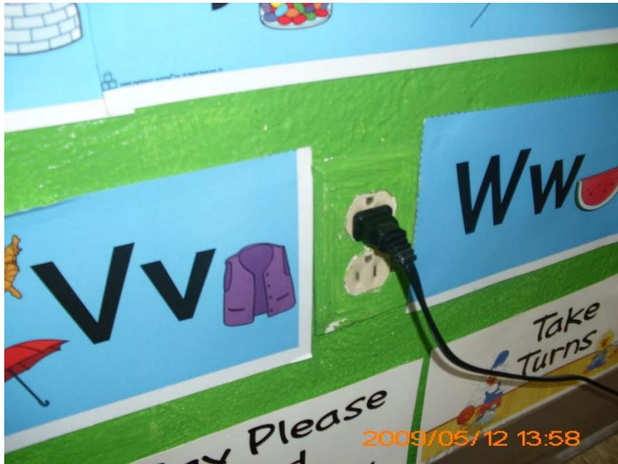
**Photograph 1 – Taken at the Bartow County facility on 5/12/09 showing an electrical outlet without a protective cap.**
