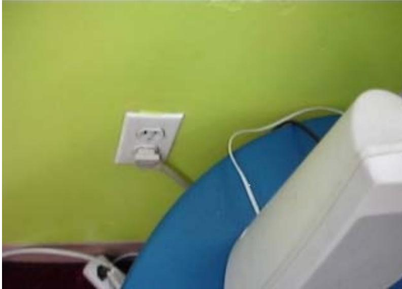
**Photograph 1 – Taken in a classroom on 7/13/2009 showing an uncovered electrical outlet.**
